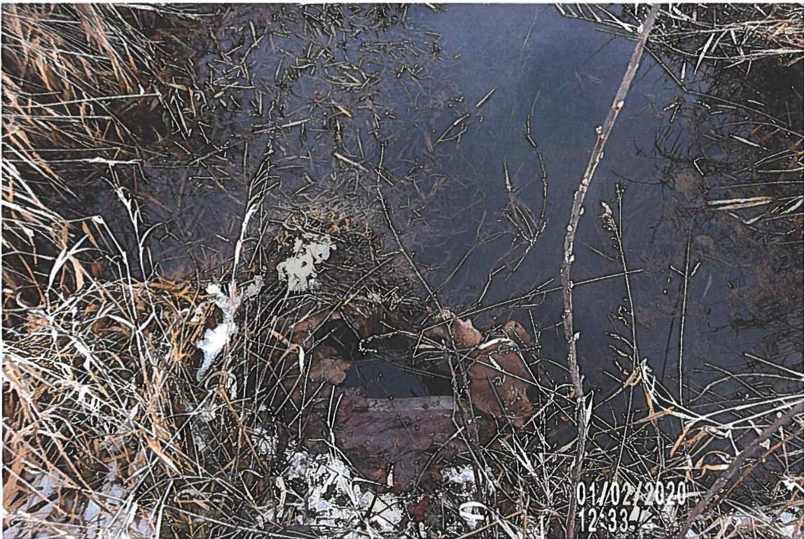
PICT# 2619 TOP VIEW OF MANGLED 30" CMP OUTLET ON N.E. SIDE
